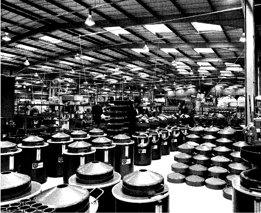
Figure 3.7.2 Factory lighting of correct illuminance, free from shadow and glare, making use of high pressure discharge lamps. (Courtesy Thorn Lighting Ltd)
