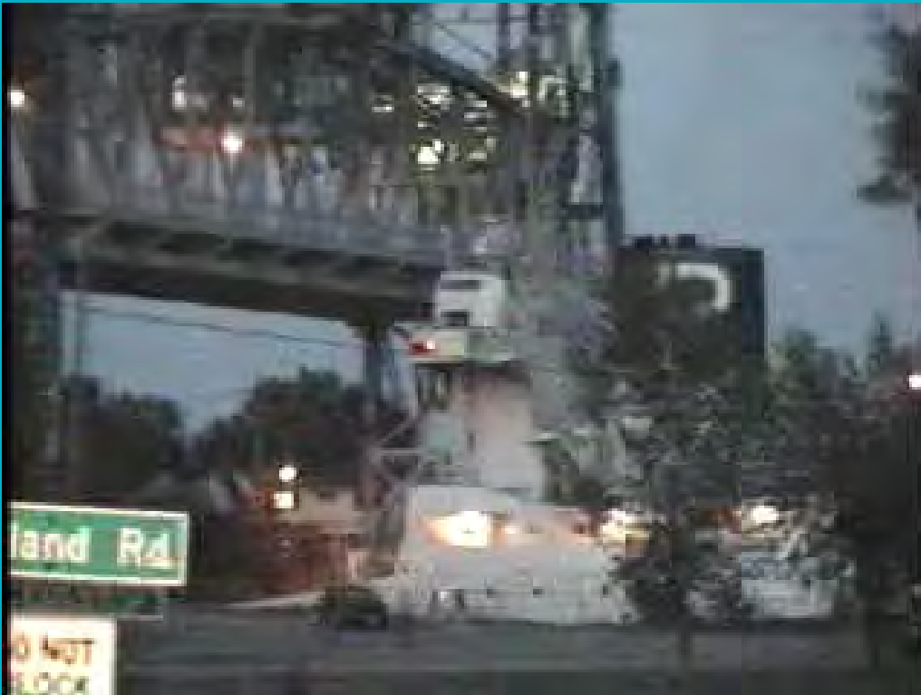
Windoc hits Welland Canal Bridge - August 11th, 2001
